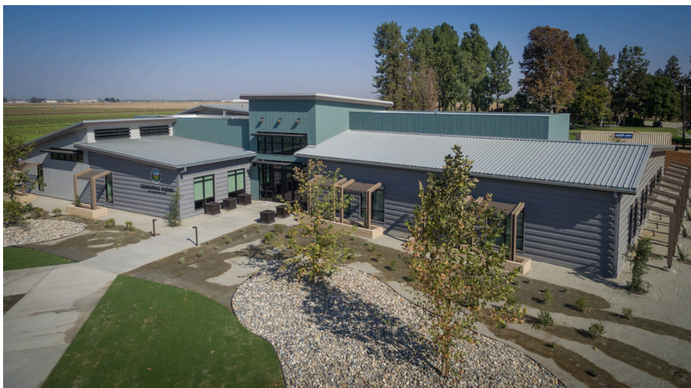
Grimmway Farms Modular Building in Arvin, CA by JTS Modular
